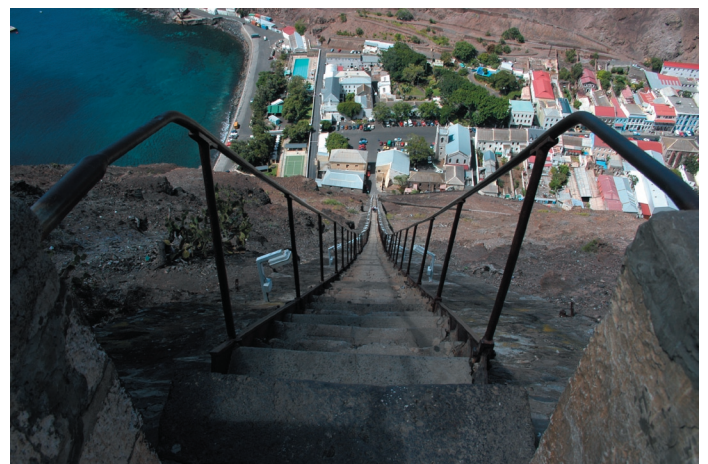
Jacob’s ladder was completed in 1829. It consists of 699 steps and the height difference is 183m.
